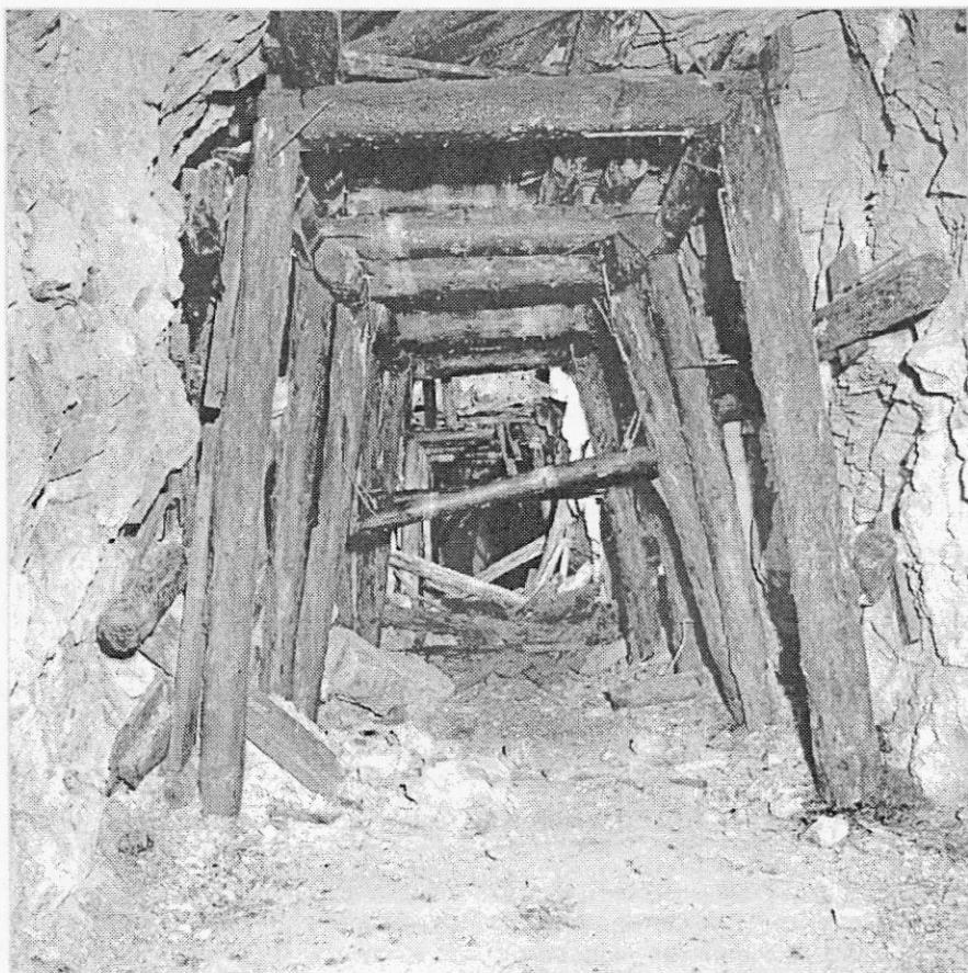
Gros Ouvrage of Flaut - Unfinished Gallery
